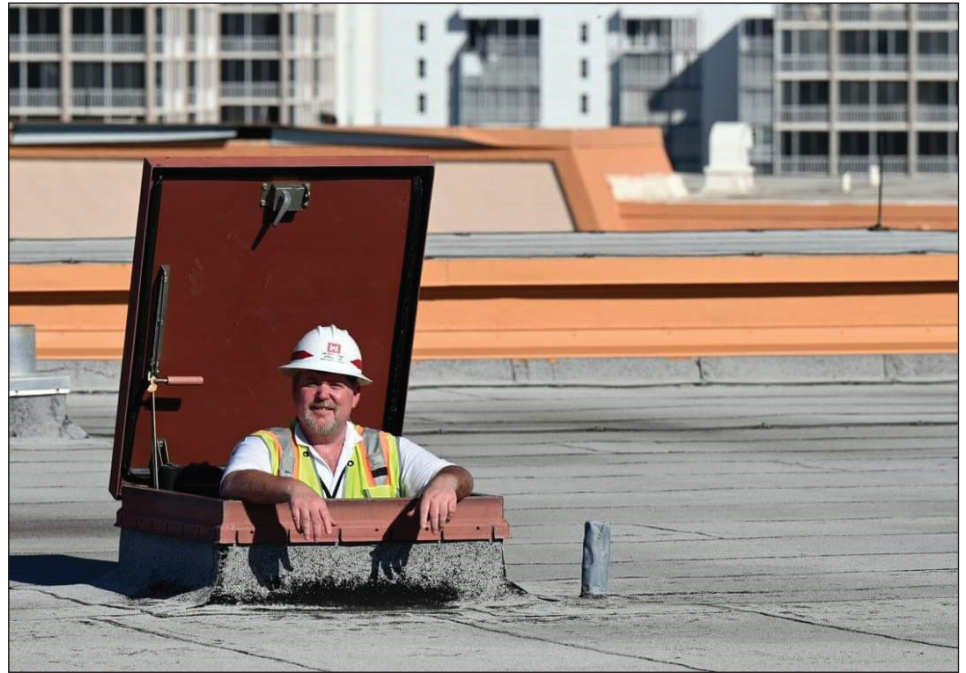
Chuck Hadley, USACE infrastructure team specialist and San Francisco District employee, looks for roof damage during a detailed evaluation safety assessment on Fort Myers Beach, Florida, Nov. 1.
